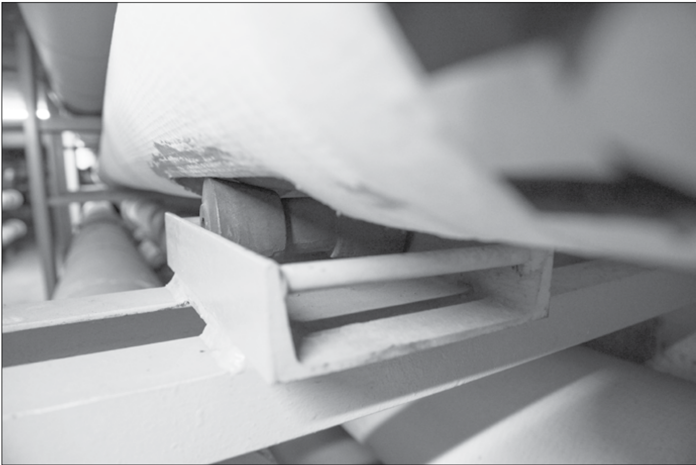
A pipe housing water and other utilities sits on a roller in the David Grant USAF Medical Center basement June 14 at Travis Air Force Base, California. Most of the pipes are fitted with seismic bracing and rollers to allow for shifting in the event of an earthquake.
